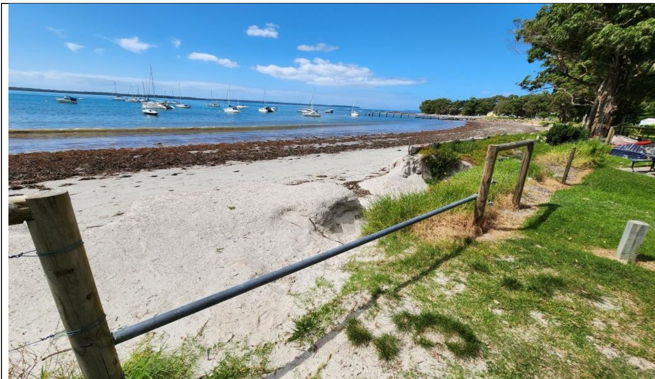
Photo 8. Eroded foreshore embankment at eastern end of Sheaffe St and recent coastal protection works
