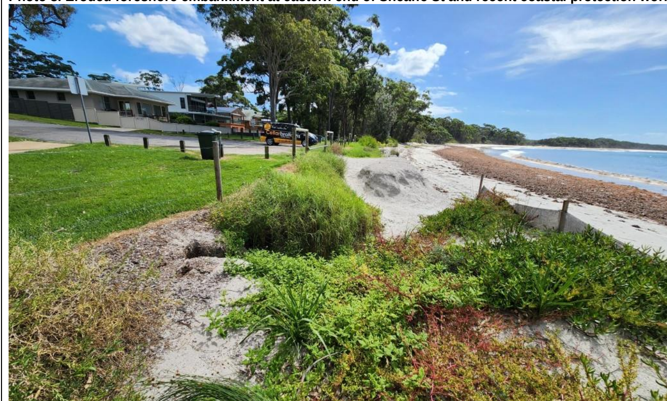
Photo 8. Eroded foreshore embankment at eastern end of Sheaffe St and recent coastal protection works
